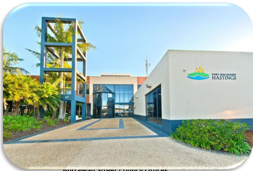
Burravan Street Council Offices
