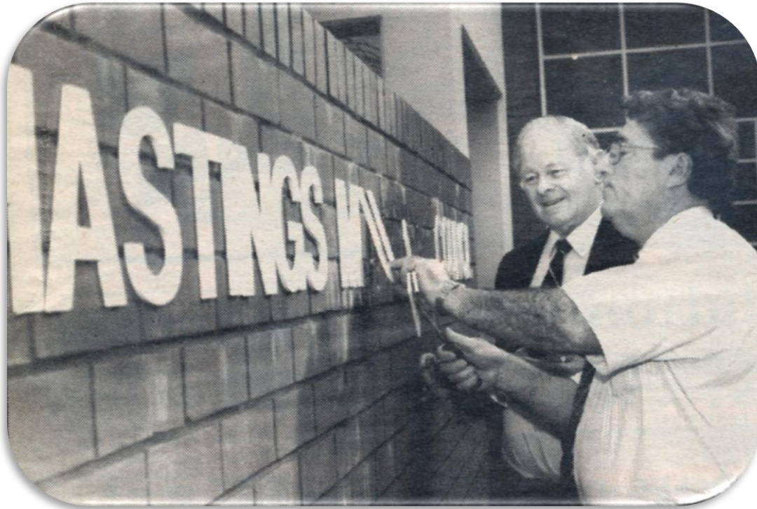
Chief Health & Building Surveyor Mr. Ron Le Pla single handedly applies a new name to the Council under the watchful eye of the Mayor Councillor Ray Cooper July 1993
