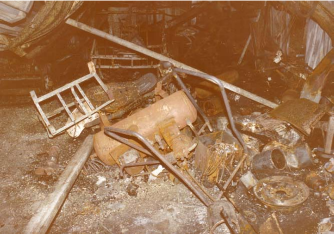
The damage suffered in the 1985 fire that destroyed the club's machinery shed is only too evident.
