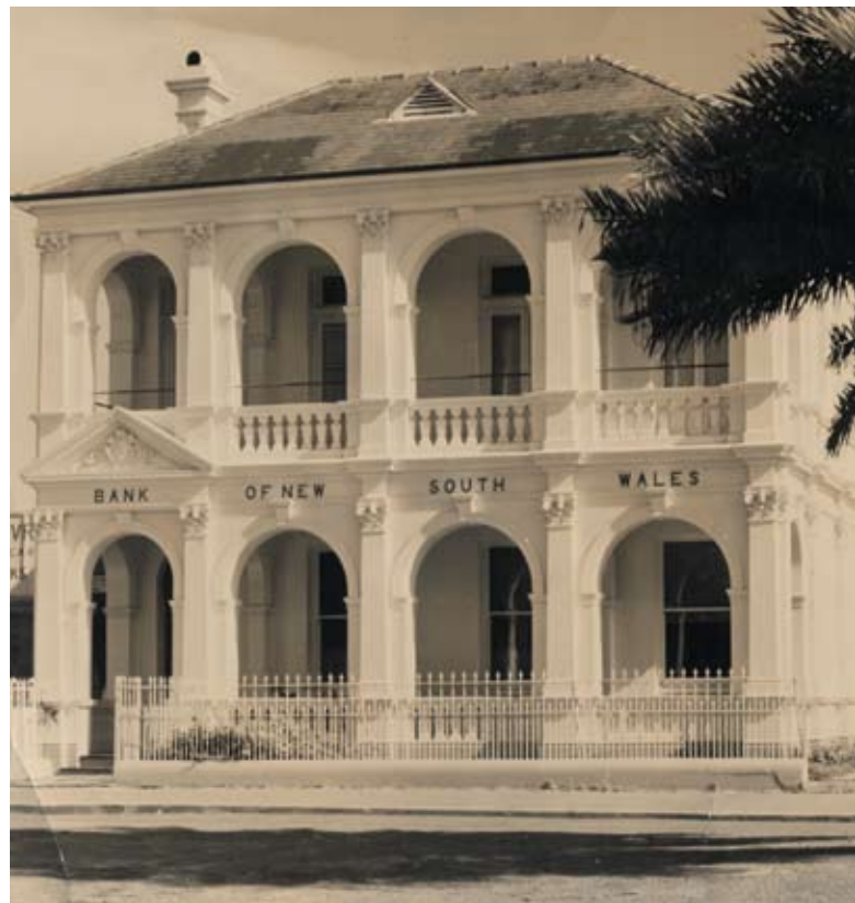
The Bank of New South Wales (now Westpac) in Horton Street...a testimony to Healey's hand-on, construction skills
