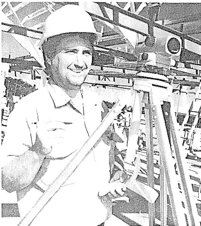
Local builder, Don Nichols, on the job setting out the brick and blockwork gridlines.
