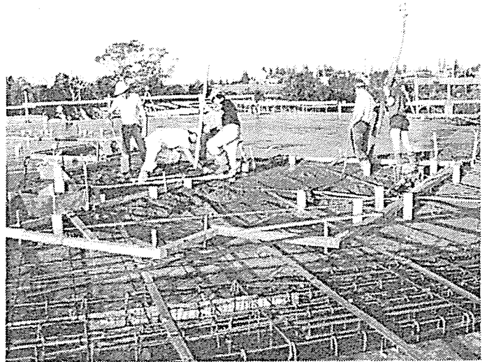
Concretors pour and level a section of the first-floor slab.
